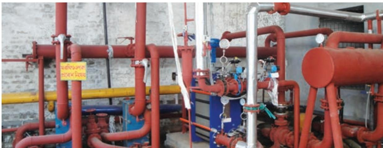
Cogeneration to recovery of heat from the Jacket Water of a Captive power Generator set for use as process heat
