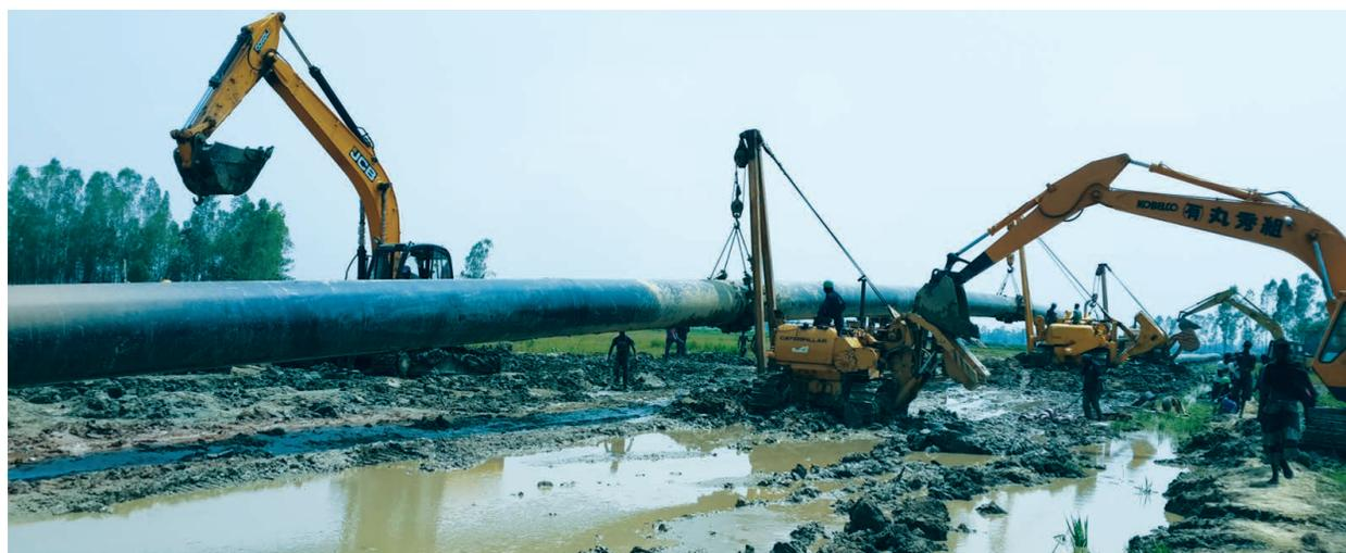
Bibiyan-Dhanua 36" diameter 137 km Gas Transmission Pipeline Project Work by GTCL
