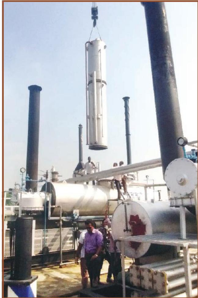
*Maintenance of reboiler of well No. 4 at Titas Field by BGFCL*
