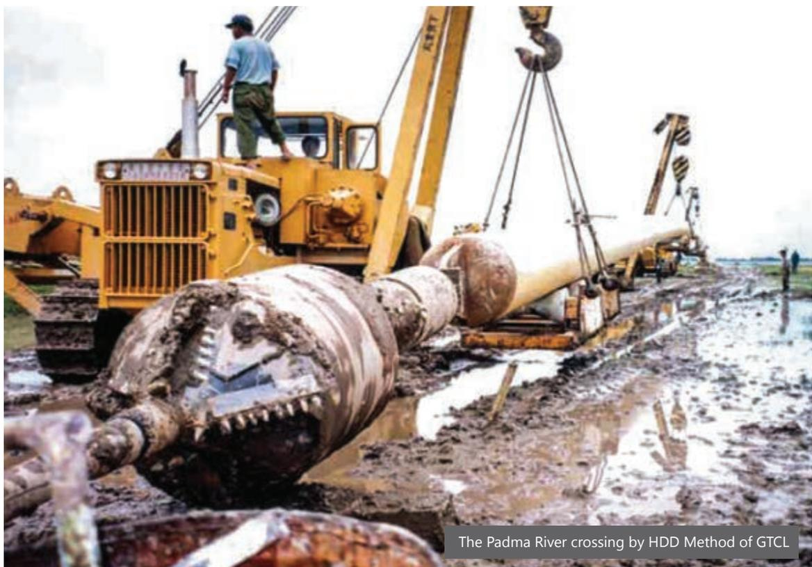
The Padma River crossing by HDD Method of GTCL
