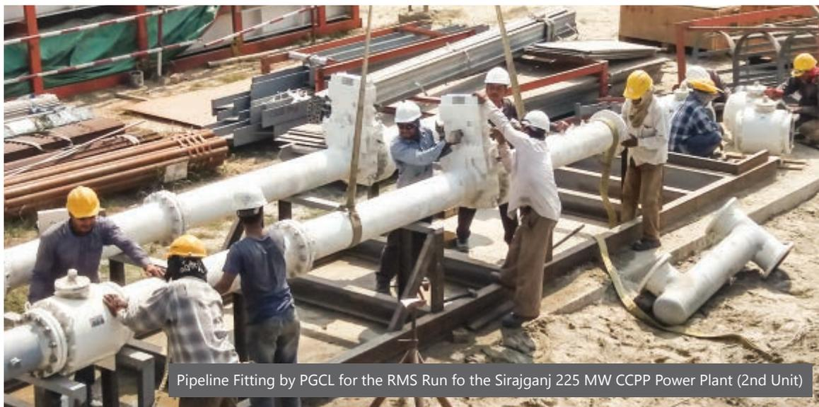
Pipeline Fitting by PGCL for the RMS Run for the Sirajganj 225 MW CCPP Power Plant (2nd Unit)
