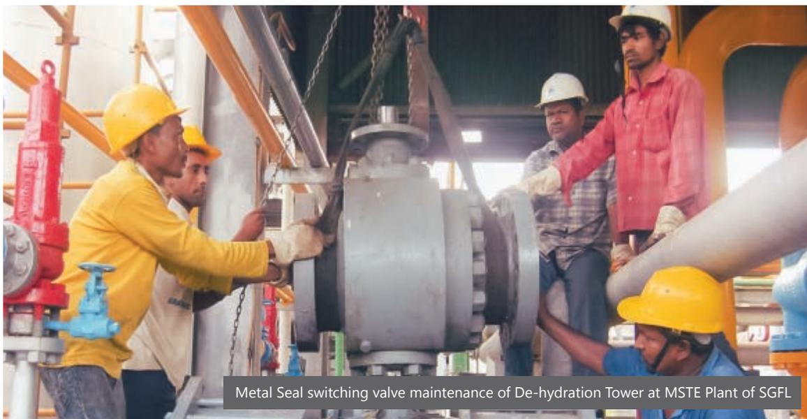
Metal Seal switching valve maintenance of De-hydration Tower at MSTE Plant of SGFL
