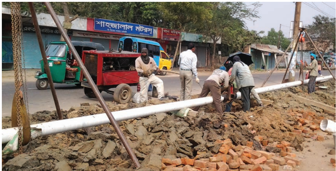
Pipeline construction work by JGTDSL.
