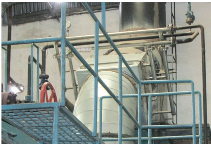
Economizer to exhaust of the boiler to recover waste heat for heating the boiler feed water
