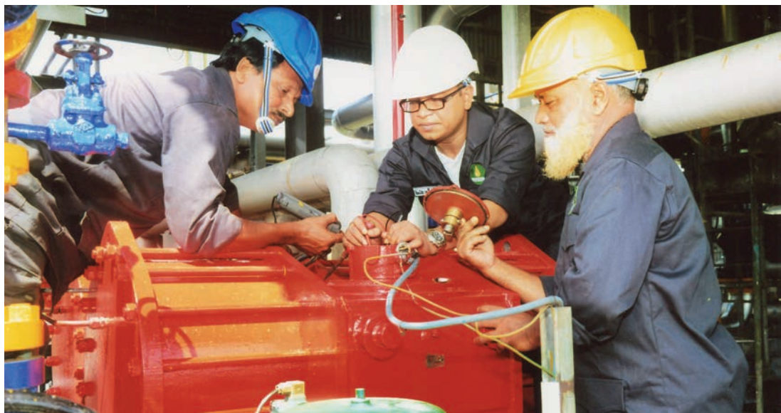
Maintenance work of Kailashtilla MSTE plant by SGFL.
