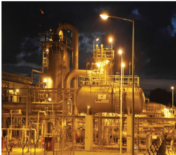
Compressor station at Ashuganj of GTCL.
