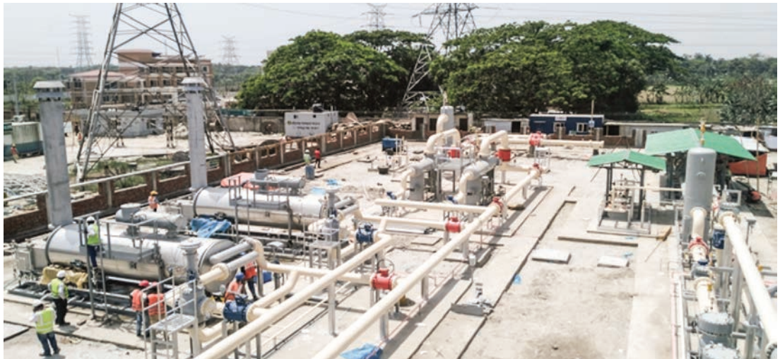
RMS at Bheramara of SGCL
