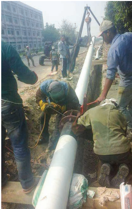
Pipeline Construction Work at Ishwardi EPZ by PGCL
