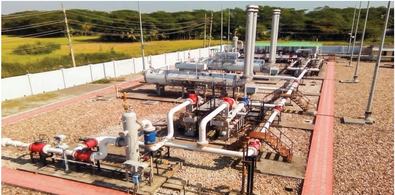
RMS of combined cycle power plant at Bhola of SGCL
