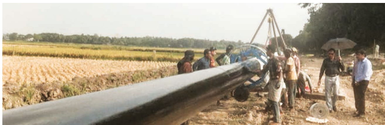
Construction of pipeline under Sreepur (Gayaran)-Joydebpur gas transmission pipeline project by TGTDCCL
