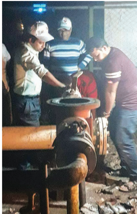
Maintenance Work of Bogra RMS by PGCL
