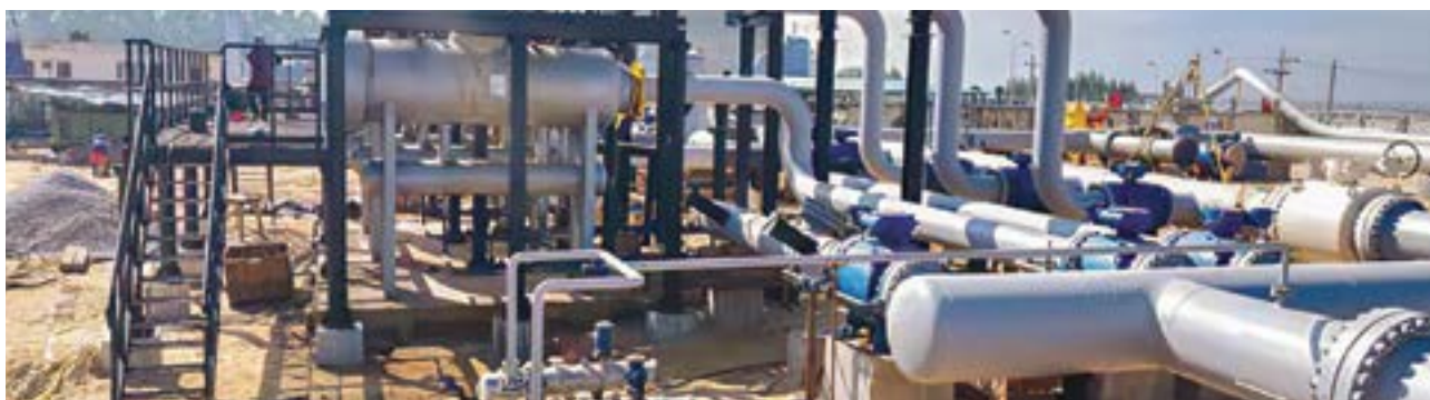
Under construction 1500 million cubic feet capacity metering station at Moheshkhali Zero Point of GTCL
