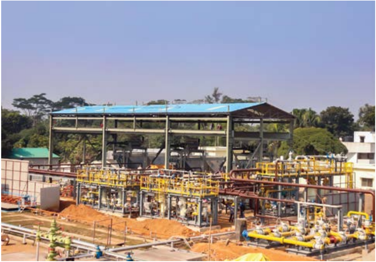
Wellhead compressor of Narshingdi Field of BGFCL
