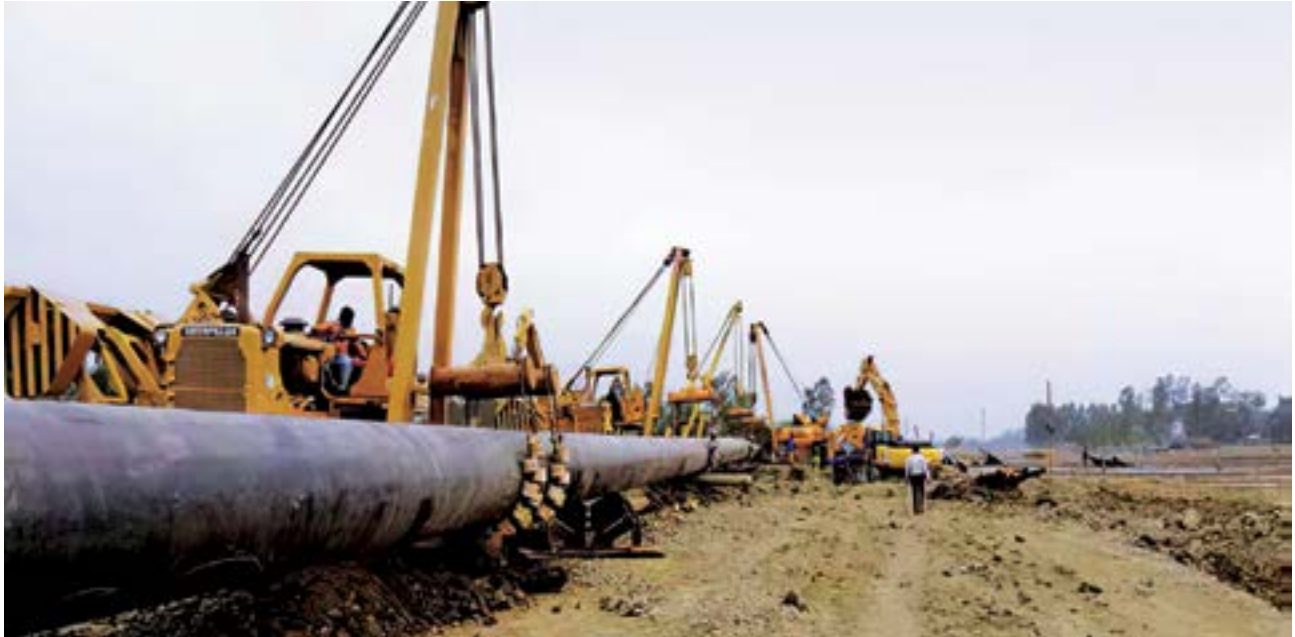
River crossing activities by HDD method under Moheshkhali-Anowara parallel project of GTCL
