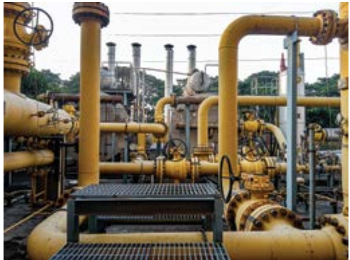
200 MW RMS at Ashuganj of BGDCL
