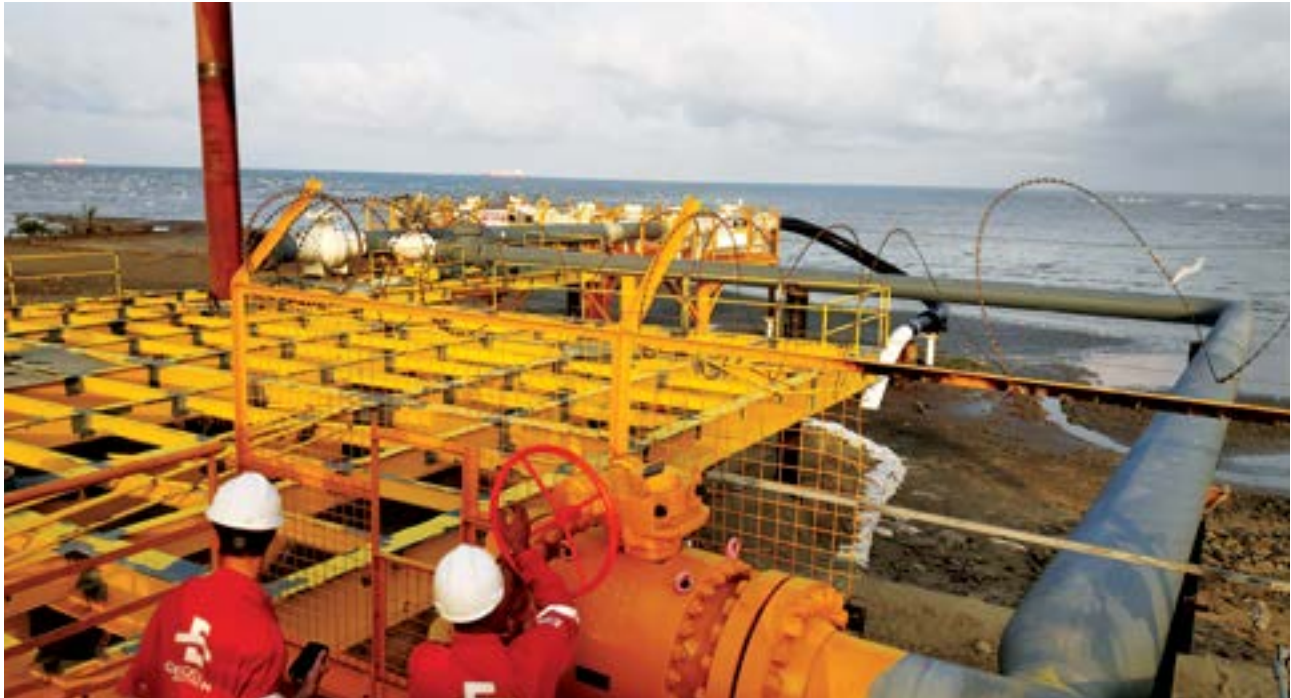
Tie-in Point Platform at Moheshkhali Zero-point Region
