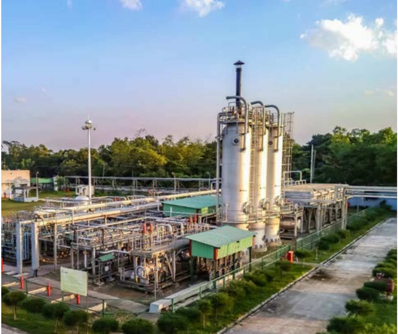
Process Plant of Srikail Gas Field of BAPEX
