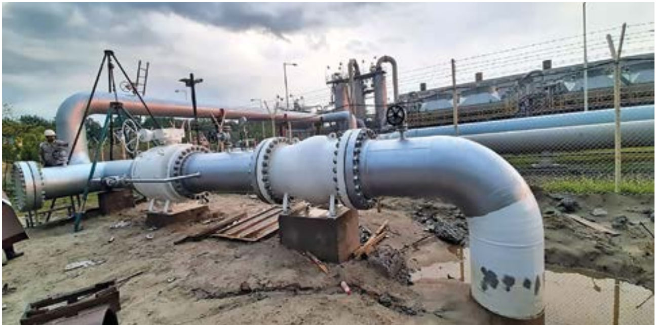
Modification activities at Ashugonj Gas Compressor Station by GTCL
