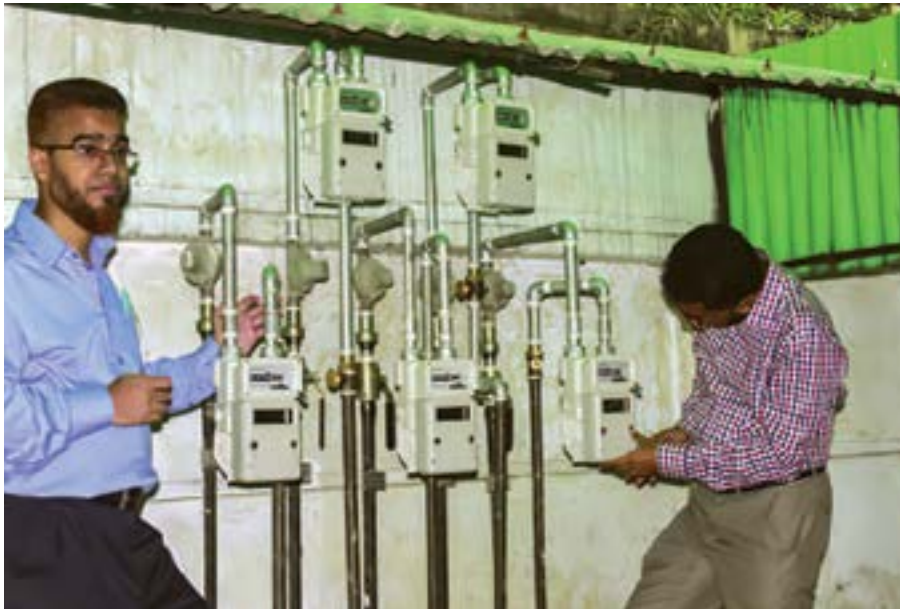
Installation of Prepaid Meter at TGTDC Franchise Area
