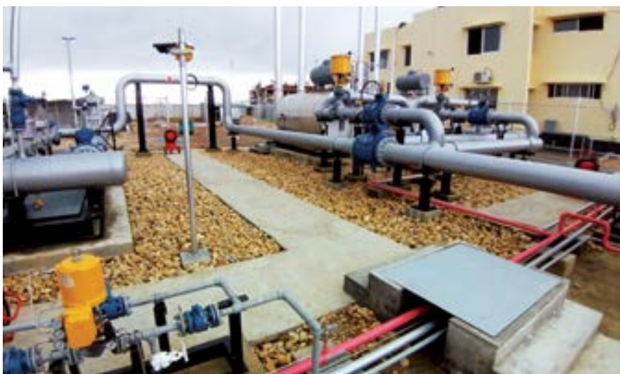
CMS of Mirasari Project of KGDCL
