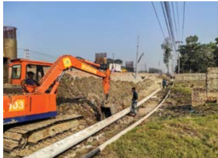
Gas Pipeline installation of BGDCL
