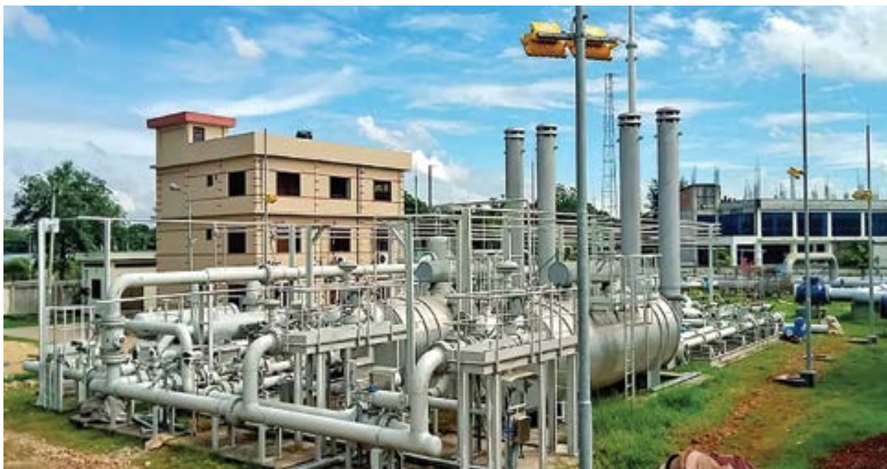
150 MMscfd capacity RMS under Dhanua-Nalka project by GTCL
