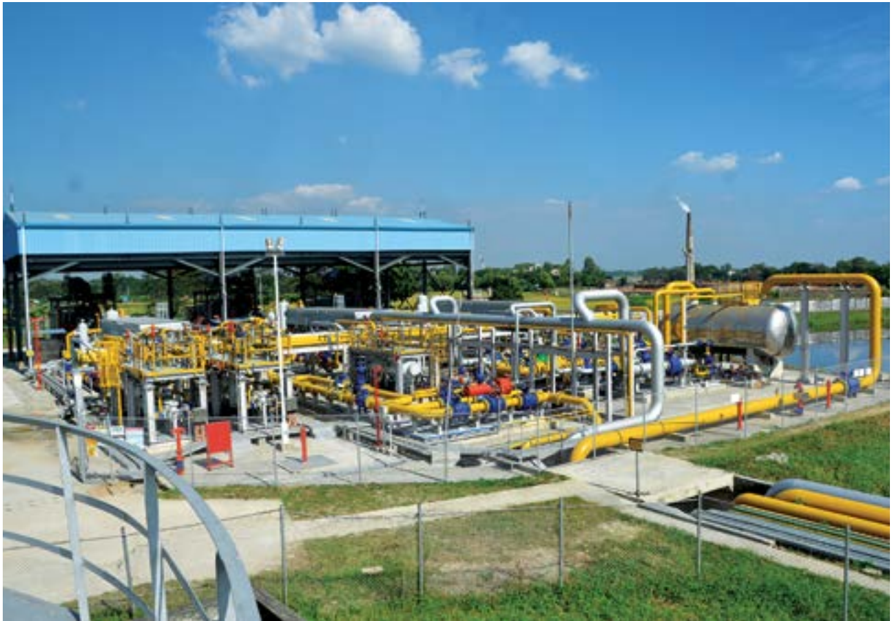
Wellhead compressor of Narshingdi Field of BGFCL
