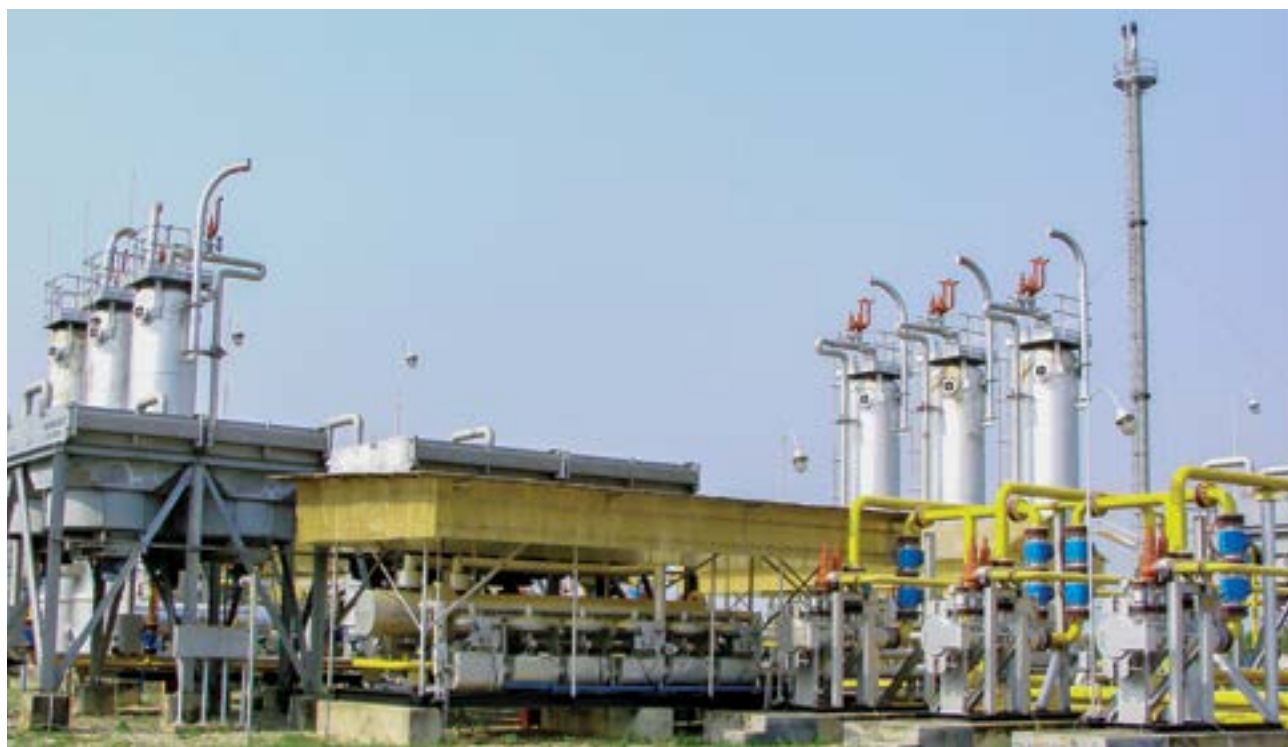
Rashidpur Gas Field Process Plant of SGFL
