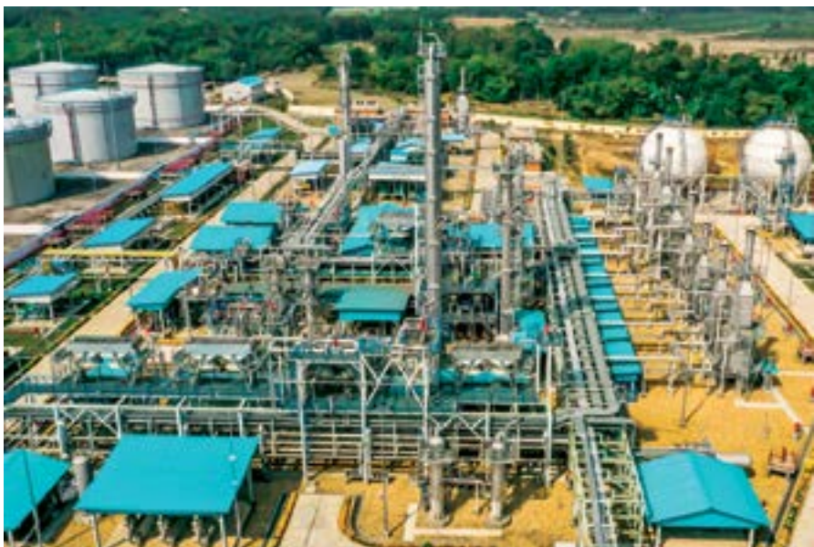
CRU Plant of SGFL
