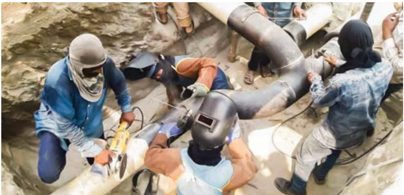
Pipeline Welding & Tie-in Connection in Bogura by PGCL
